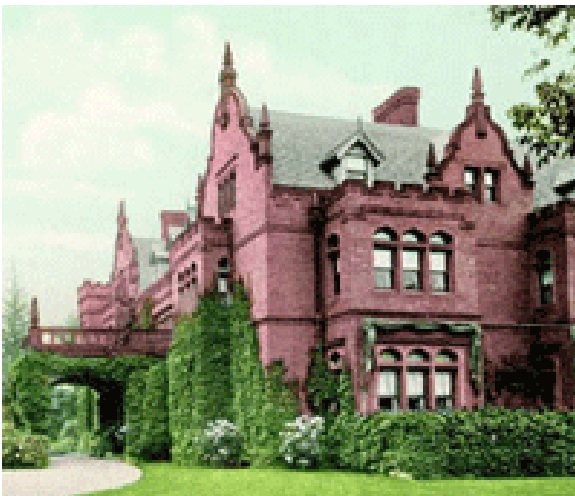
Ventfort Hall in Lenox, MA
